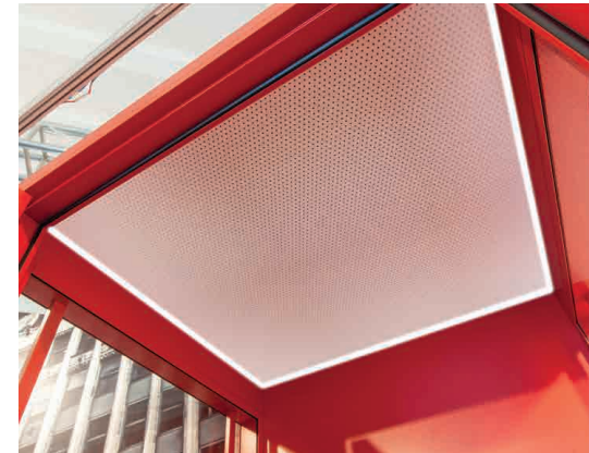
Integrated LED lighting on the perimeter of the ceiling panel.
